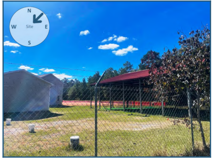
View of site from the northeast
